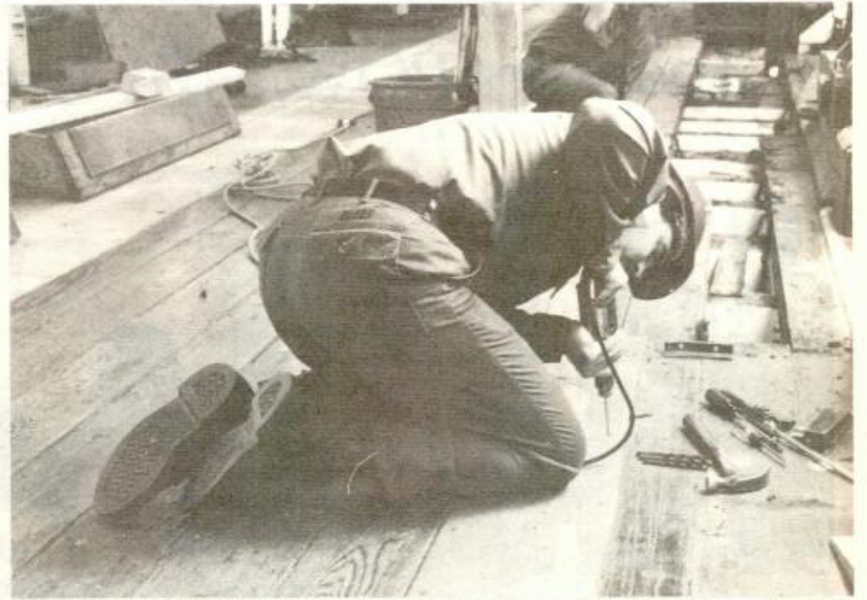
CMCN CHRIS D. ELIAS is shown drilling out brass screws in order to remove a deck plate from the main deck of USS CONSTITUTION. (photo by LCDR Vic Beck).
