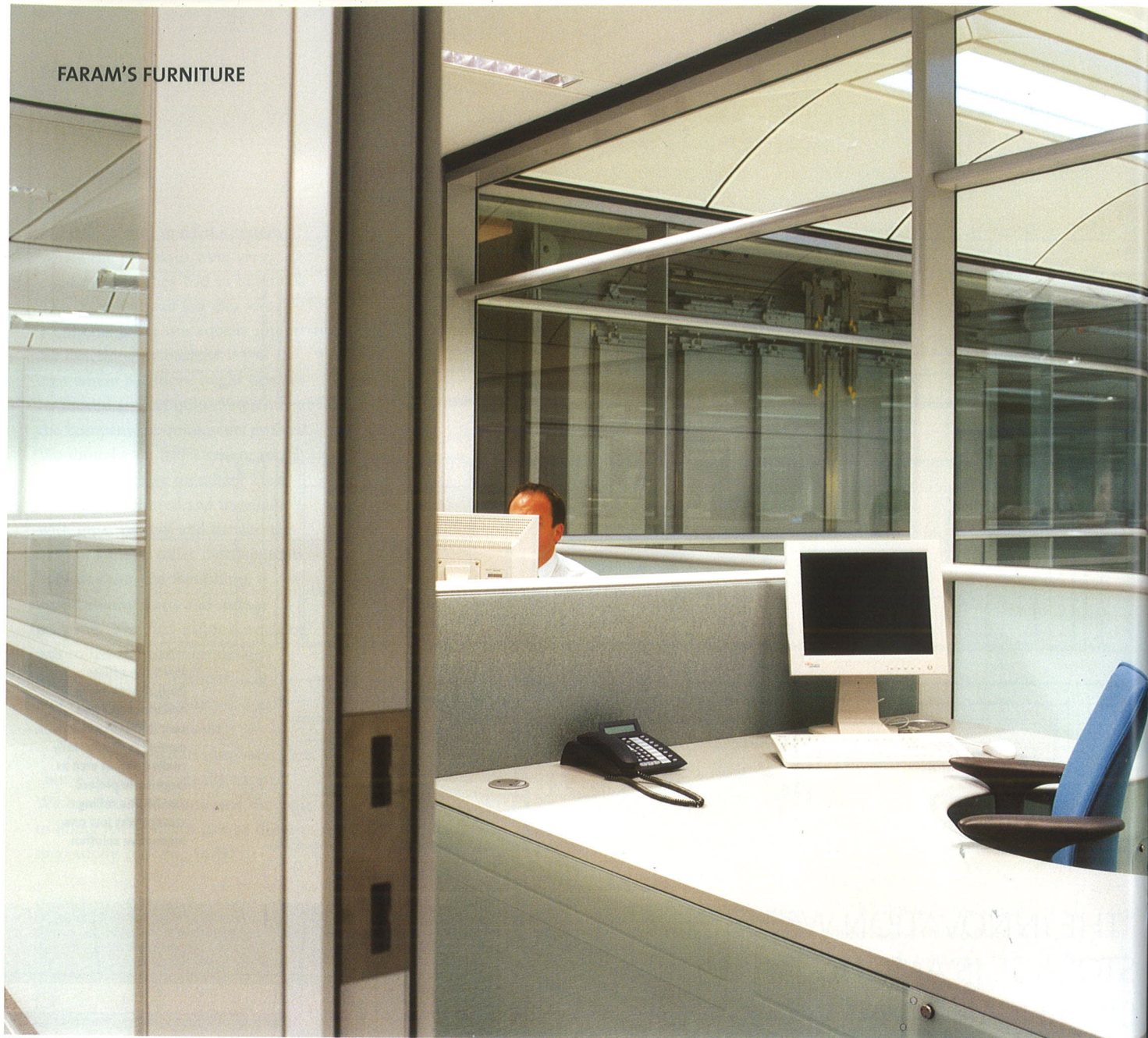
ABOVE Note that the partition glass is flush with its frame. It is bonded direct to the structure, rather than being framed by it, giving the offices a clean, glazed look
