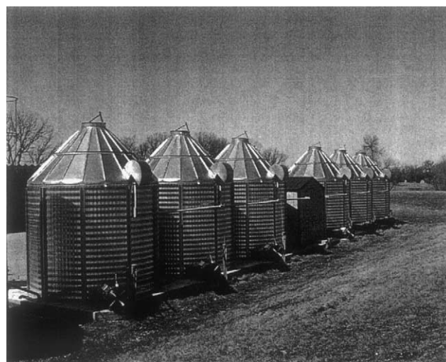
Fig. 2. Corrugated steel, flat-bottom bins at Cereal Research Centre Farm (28 tonne capacity).
