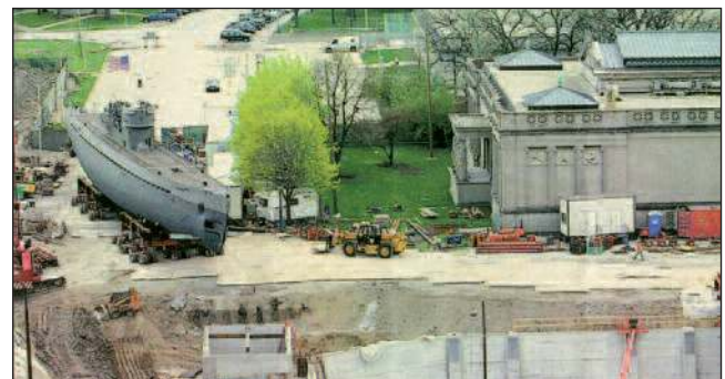
to the 'Windy City' taking over a month. However, exposure to the elements over the following 50 years resulted in considerable deterioration so a $35 million project was mounted in 2004 to move the boat to a specially-constructed, climatically-controlled underground facility.
