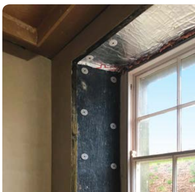
FOT. ENVIRONMENT INSULATION
