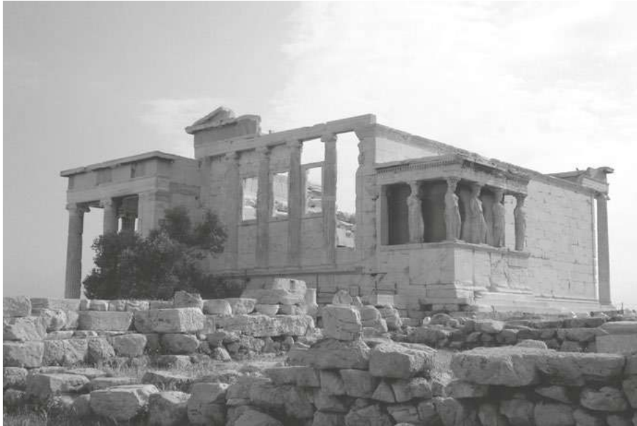
Fig. 43: The 'Periclean' Erechtheion and the olive tree.
