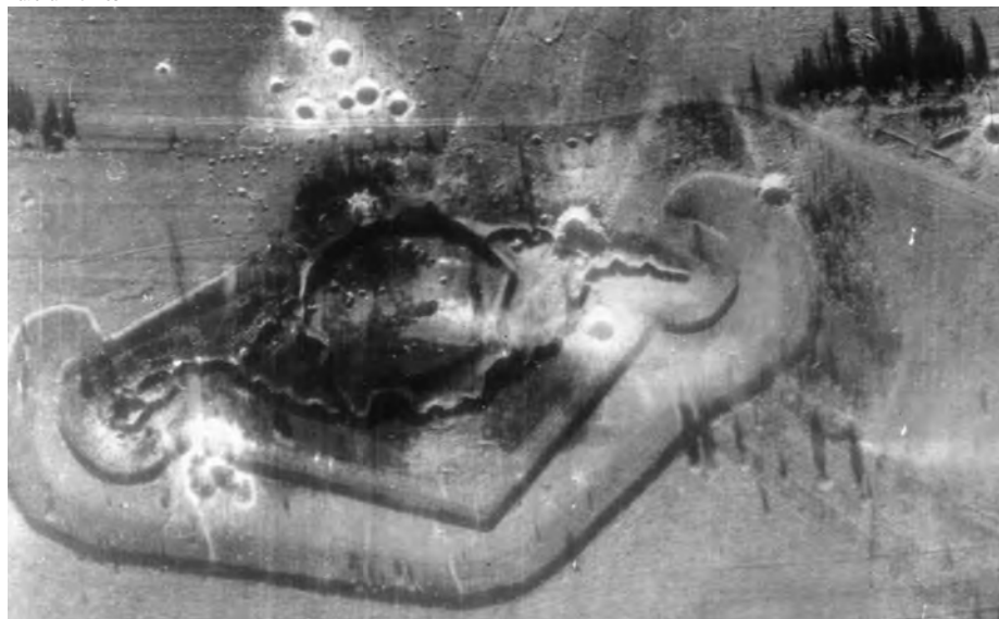
ABOVE: Although the bomb craters look impressive, the walls of Fort Driant were barely dented by American air power. BELOW: After the battle, the reinforced concrete walls of Fort Driant show the effects of shells and bombs but have not been breached. The fort did not fall until December 8, 1944.
