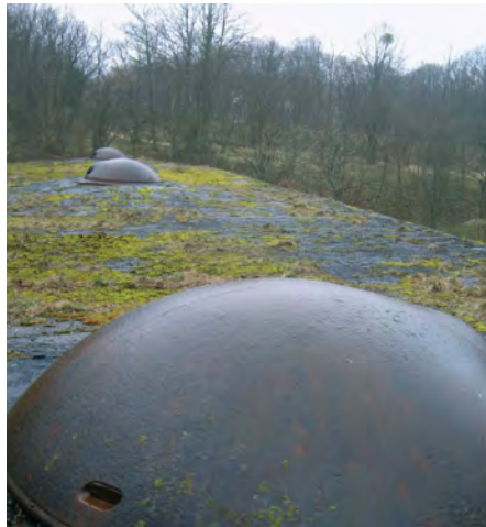
ABOVE: The steel cupolas of Fort Driant as they appear today. Although derelict, the fort is still used by the French army for training purposes.
