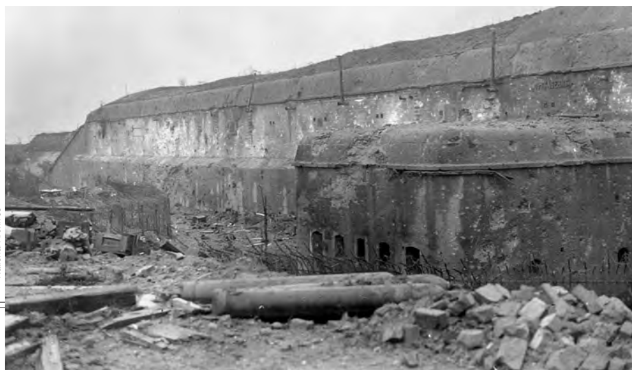
ABOVE: Although the bomb craters look impressive, the walls of Fort Driant were barely dented by American air power. BELOW: After the battle, the reinforced concrete walls of Fort Driant show the effects of shells and bombs but have not been breached. The fort did not fall until December 8, 1944.
