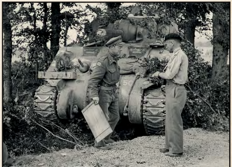
BELOW: Major General George 'Pip' Roberts DSO, MC (right), commanding 11th Armoured Division, with Brigadier Roscoe Harvey DSO, of 29th Armoured Brigade talk in front of Roscoe's Sherman command tank (note extra aerial on the front hull for the additional No.19 wireless, but retained main armament), in a Normandy staging area, 15 August 1944. (HMP)
