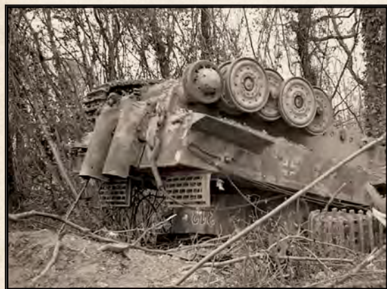
ABOVE: Tiger 313 of Schwere Panzer-Abteilung 503. Nearly 60 tonnes impressively but brutally flipped by bombing prior to Goodwood. Tiger 313's servcability however, is in question, as earlier photos show 313 took a powerful, but non-penetrating, hit to the side, leaving a deep fist-sized dent.
