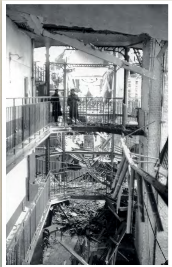
ABOVE The damage inside the prison.
