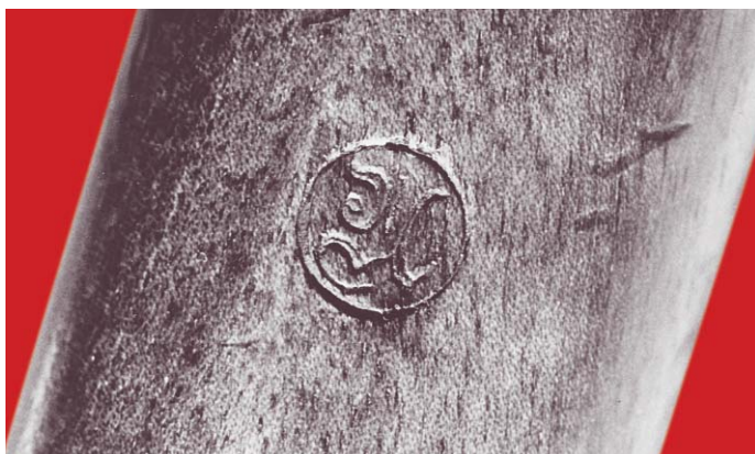
View of the wrist of a "C"-series Mauser Rifle, showing the unusual circle marking as found on the receivers of many ZAR and OVS Mauser rifles. (John Wall collection, photo by John M. Leone)
