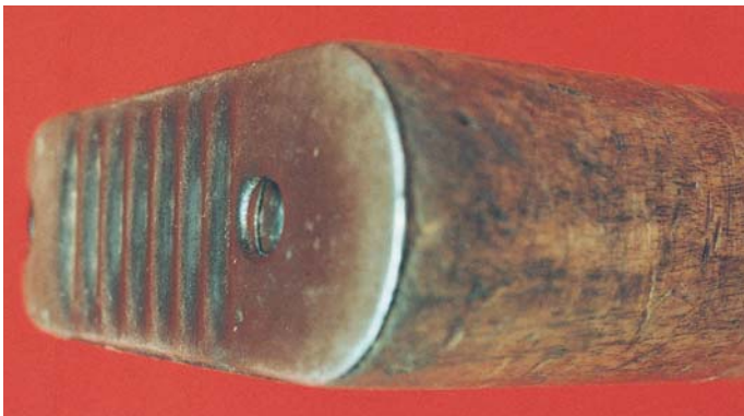
The "corrugated"-style buttplate used on the Haitian FN Model 24/30 Short Rifle.
