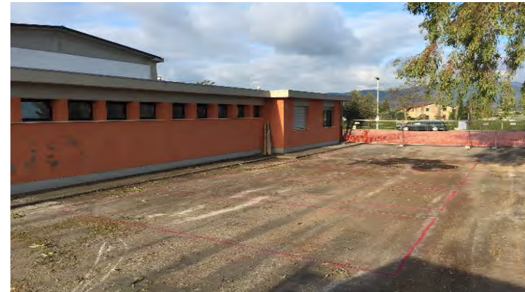
State of the building before the work
