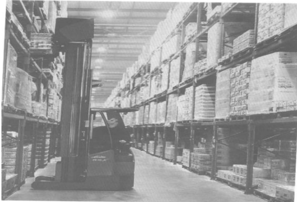
Adjustable pallet racking, being served by reach truck
