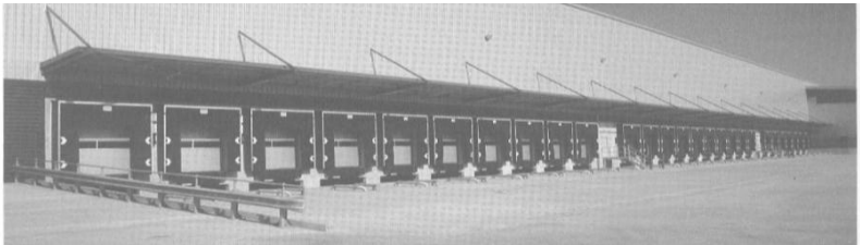
Raised dock loading bays
