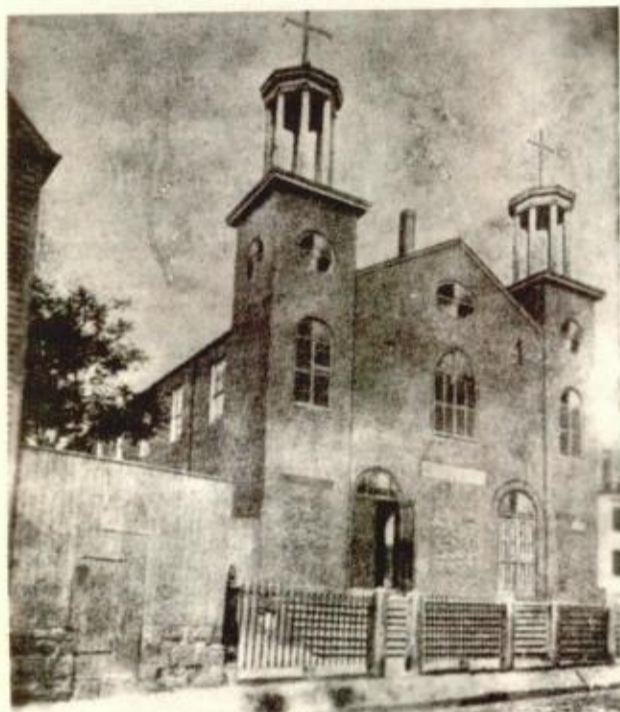
ST. MARY'S CHURCH on Richmond Street, which is now Old Rutherford Avenue, was used by the parish from 1829 to approximately 1888. There were galleries on three sides, the interior showed patterns and scrolls in fresco on the walls and ceiling and had several paintings.
