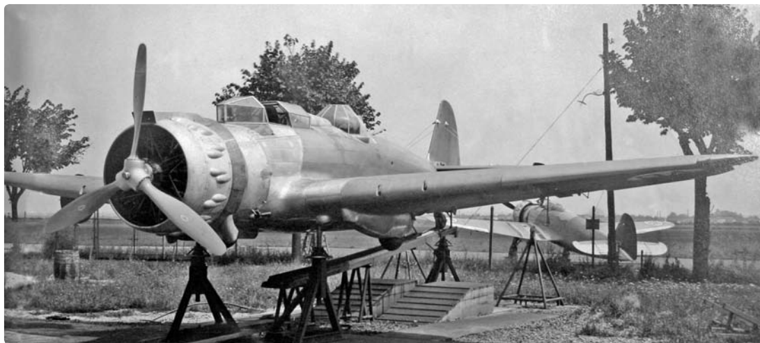
ABOVE With a single-seater in the background, one of the FACH's three turret-equipped Ba.65s has its compass swung at the Breda works in Milan before delivery. Some 25 Ba.65s were acquired by the Royal Iraqi Air Force in 1938, the majority being fitted with the same Type M turret, which significantly hampered the type's performance.
