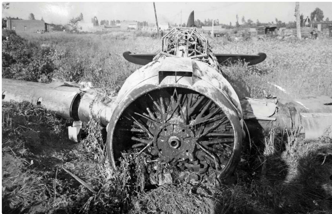
ABOVE The charred remains of Ba.65 No 5 (c/n 64186), which came to grief after engine failure during a gunnery practice flight on October 31, 1939. Thankfully, the pilot, Capt Hernán Lopez Angulo, was one of the more experienced FACH pilots and managed to execute a skilful forced landing in a field at Maipú, near El Bosque AB. The aircraft was destroyed in the ensuing fire, however.
