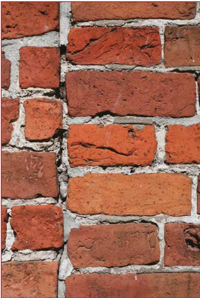
▲ Red fire bricks are best for making a kiln.
