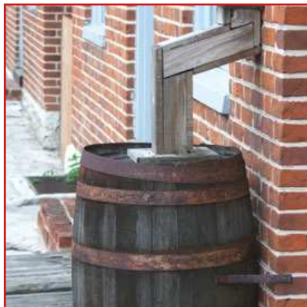
▲ Rain barrels can be made from any large bucket. It is especially convenient to have a spigot coming from the bottom of the bucket so you can fill smaller containers with water as needed.
