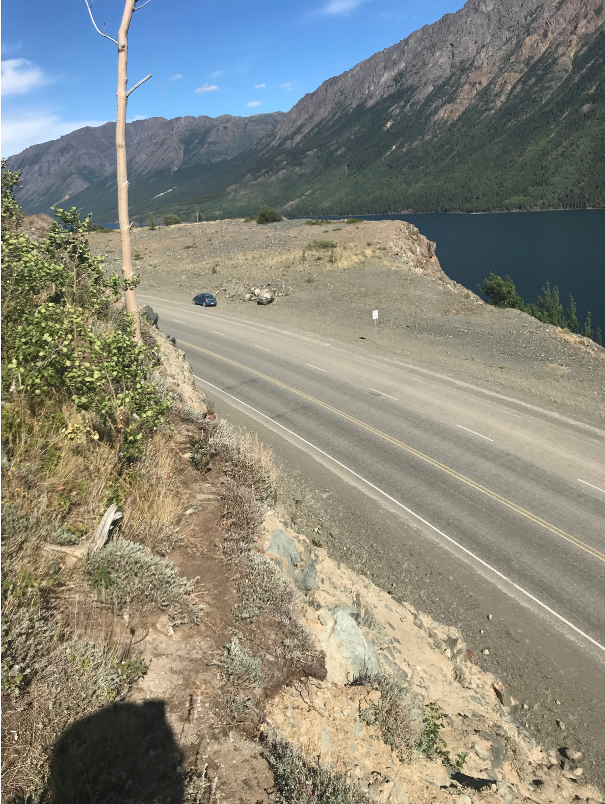
Figure 6 Gravel pullout at Crossing 2 as viewed from a mountain goat trail above the highway.
