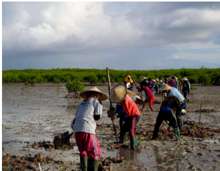
An example of community-based ecological mangrove restoration (CBEMR), Tanakeke Islanders hand digging 1.5 km of tidal creeks in disused shrimp ponds to restore natural hydrology. PHOTO: YUSRAN NURDIN
