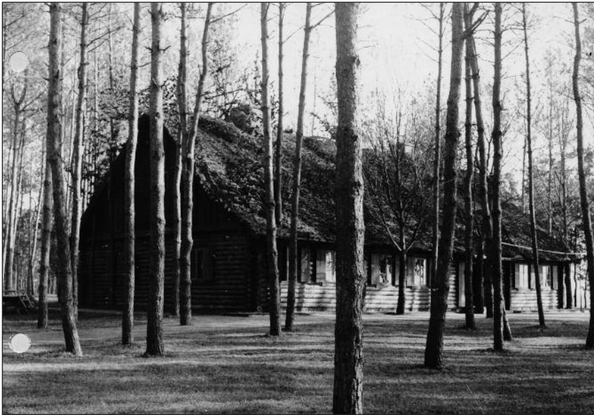
Diagonally across the meeting square from the Kasino/Teehaus, close by the southern edge of Sperrkreis I, stood House No. 11, Hitler's private lodge [17]. Measuring 19,5 by 8,5 metres, it had only one entrance and comprised eight rooms. Hitler lived here accompanied by his personal valet SS-Obersturmführer Heinz Linge. Hitler's office was at the far end. Note the camouflage netting on the roof and the seating area to the left of the house.
