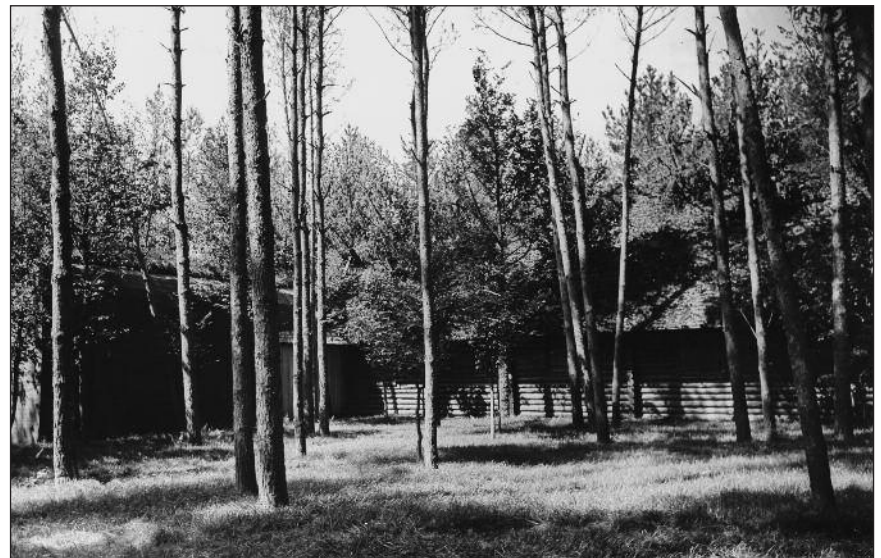
Built against the rear of the house was Hitler's personal air raid shelter, seen here on the left. Accessed through a door direct from his office, it had roof and walls two metres thick and an internal space of six by six metres.
