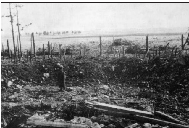
Left: The remains of Hitler's private bunker seen from the foundations of his house. This picture clearly illustrates how close the bunker was to the edge of the forest. Very few items of interest were found by the Soviets, the NKVD report detailing
