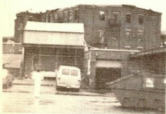
AMERICAN PAPER BOX COMPANY in Sullivan Square faced extensive damage from the storm as the winds lifted off the roof of the structure.
