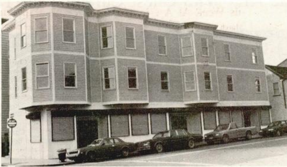
142-144 BUNKER HILL ST. must have city Board of Appeal grants its approval for serious code violations corrected before the renovations.
