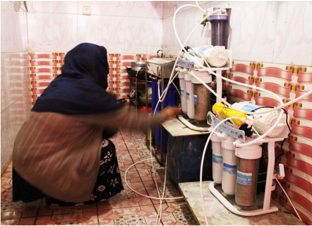
Maryam's water purification machine which fills the bottles outside through a pipe
