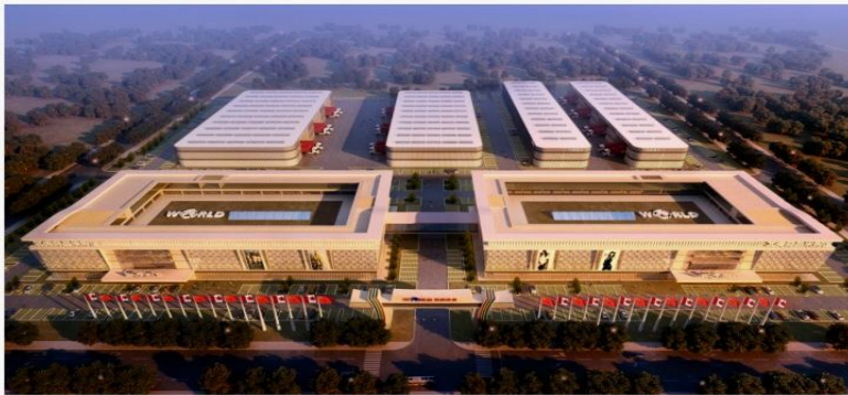
Joint Canada-China World Commodity Center under construction in south Surrey, BC
