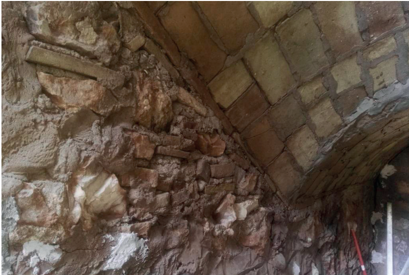
Figure 8: Rammed wall and timbered vault in the antechamber of the Camí d'Onda Air-raid Shelter in Borriana, Spain, picture by Ivan Cabrera i Fausto.
