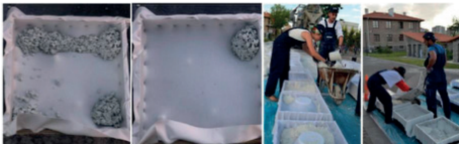
Image 15: Concrete casting process of the fabric formwork-based design.
