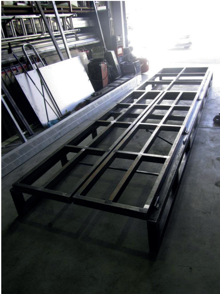
Figure 12: Constructive process of the steel structure of the transformable bench for the access of the Camí d'Onda Air-raid Shelter in Borriana, Spain, picture by Ivan Cabrera i Fausto.
