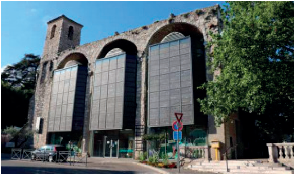
Figure 7: PV panel integrated façade of Tourist office of Alès (Heinstein, Ballif, & Perret-Aebi, 2018)
