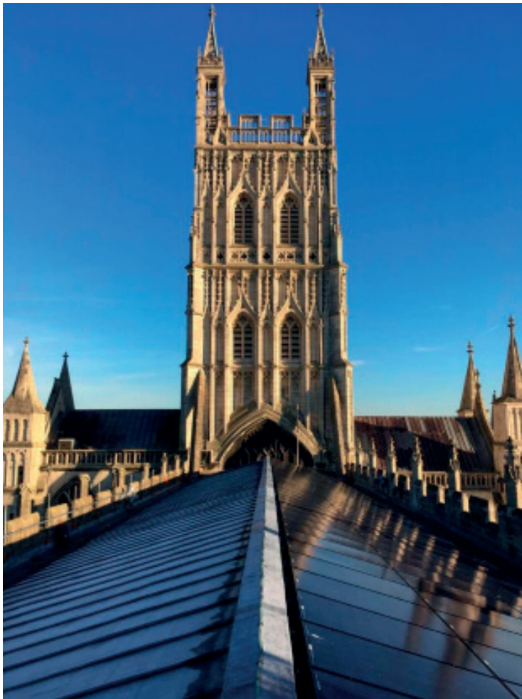
Figure 10: Photovoltaic panels on top of the roof of Gloucester Cathedral (mypoweruk.com)
