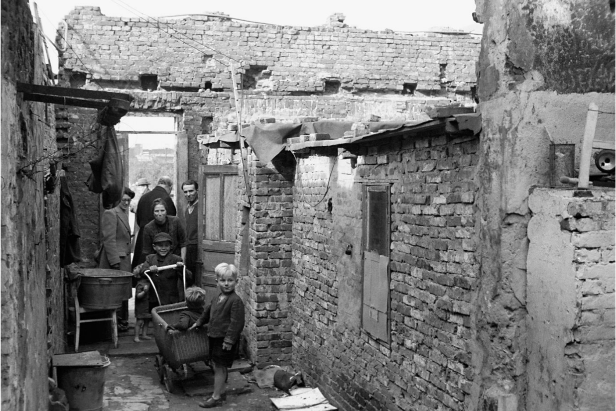
Life amongst the ruins: For the rest of the war, and for years afterward, families were forced to live in the most basic of conditions wherever they could find shelter. (Denkmalschutzamt Hamburg)
