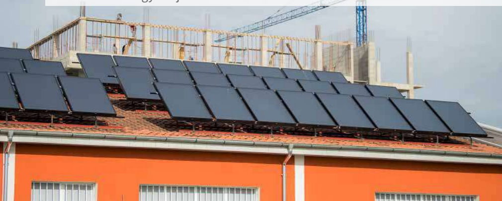
The Orthopedics Clinic of the main hospital in Pristina is one of the first 32 public clinics and schools that have been upgraded with energy efficiency and renewable energy investments as part of the WBG’s Energy Efficiency and Renewable Energy Project in Kosovo.
