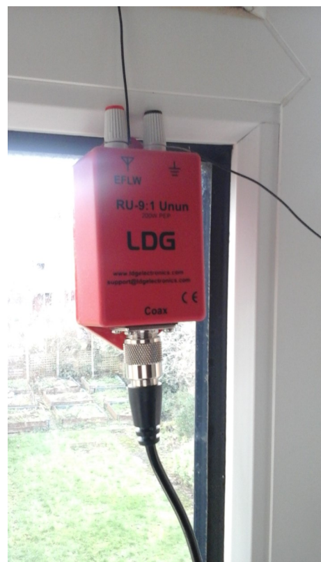
53ft of wire from the 9:1 UnUn with the counterpoise earthed to the copper water pipe
