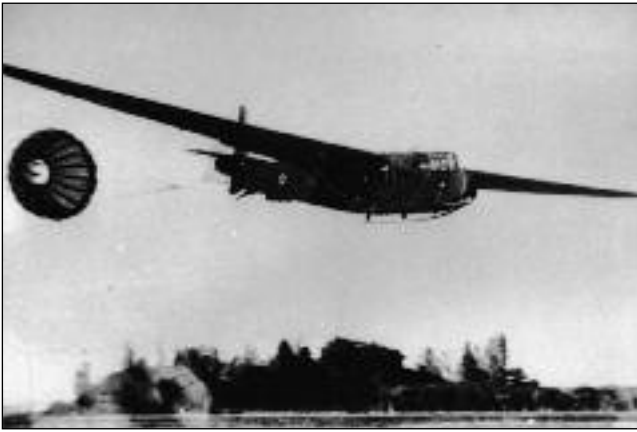
Immediately in the wake of the paratroopers, the glider force arrived, all the aircraft being fitted with parachute brakes to shorten their landings.
