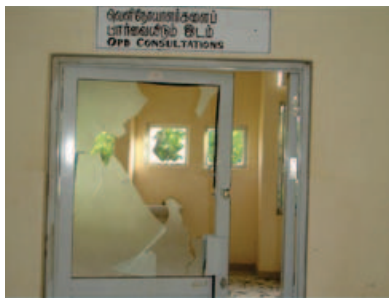
Figure 3.5 Artillery shell attack on Kilinochchi General Hospital, December 2008
