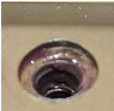
Figure 3: Permanent Chassis Deformation after 30 in-lbf install
