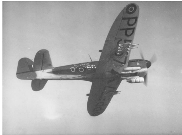
Fairey Firefly FR.I of 816 Sqn . Overflying Malta. The under fuselage Radar, for use in the anti submarine role, identify it as a FR.I. J I Agnew
