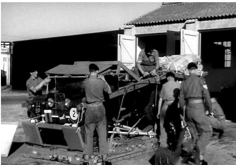
Early Land Rover on an MSP parachute dropping platform. cheshire steve
