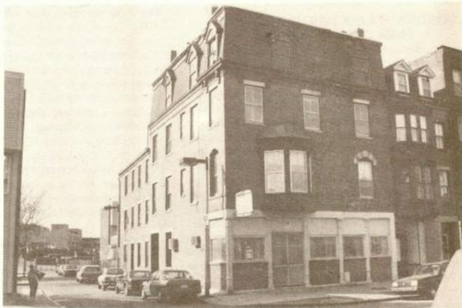
THE FORMER Charlestown Co-op Bank building on 250 Main St. and 1-3 Phipps st. are expected to house seven apartments and one retail space. High Pharmacy owner Carmen Merlino has proposed to redevelop this historic building.
