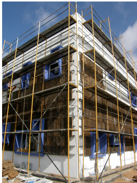
Image 18 - Cork-oak and Cork Observatory / Coruche ventilated cork facade setting up
