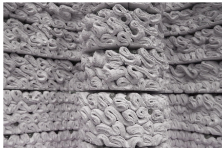
Image 8 - Firewall: 3D Concrete printing, by Bekkering Adams Architects and TU/Eindhoven, Photographer: Bekkering Adams Architects
