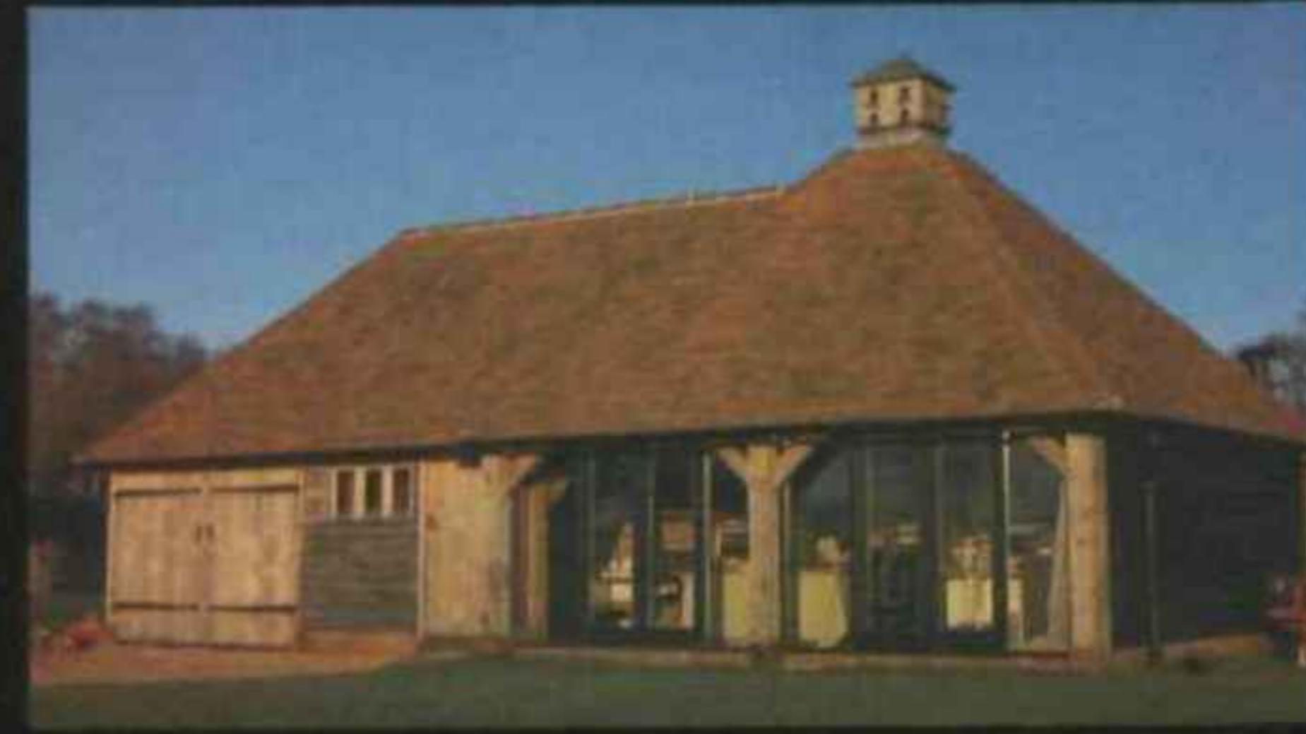
GARAGE & OFFICE COMPLEX No. 380
