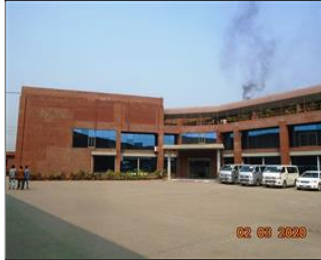
External photo(s) of the production unit(s) Factory building 1.JPG
