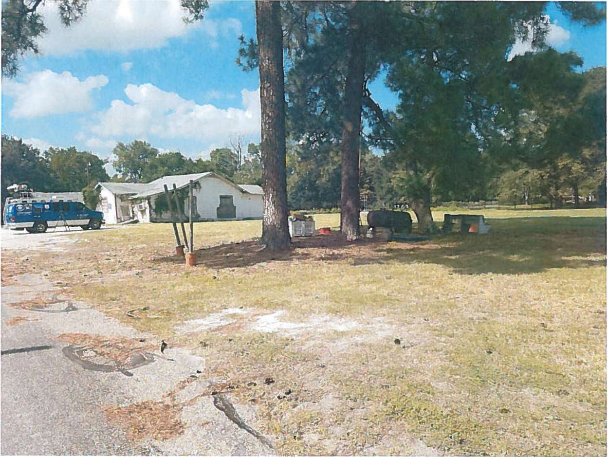
Abandoned Sandbranch Community Center for proposed pump station or lift station site
