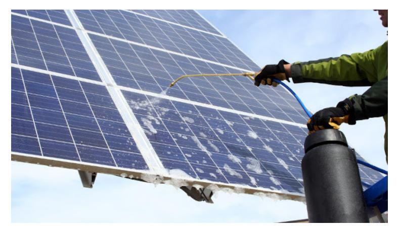
**Step #02** - Spray each panel from top to bottom; Move onto the next one until all four have been cleaned through this method; opt for an electric pressure washer option as well.
