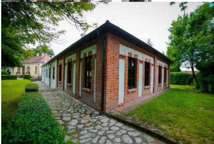
Figure 28. Position of the ambient subunit within Zone 1 of the Scope of the Competition; Figure 29. Old Assembly
