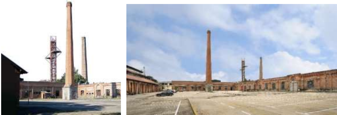
Figure 62. Old Tall Chimney
