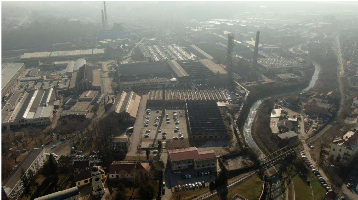
Figure 37. Panoramic view of the complex "Military-Technical Institute" and the northwestern part of the contact zone 3.1
