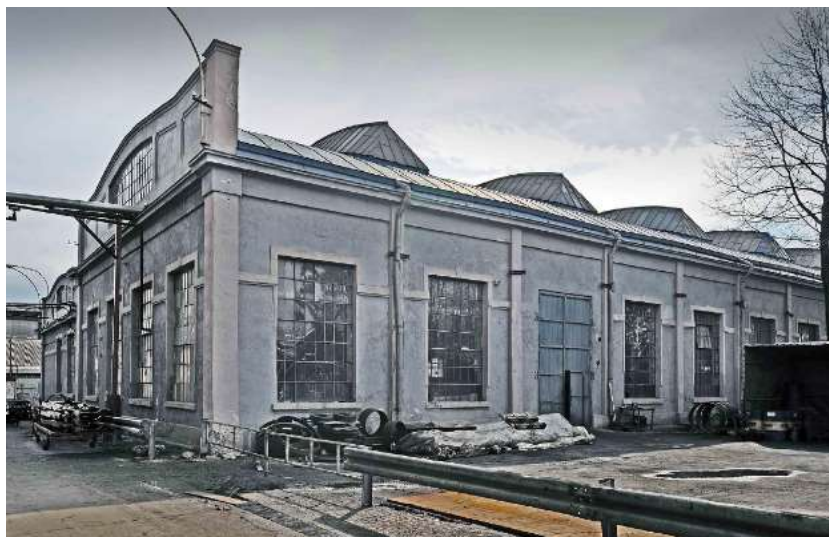
Figure 83. R.A.P. Production Hall
