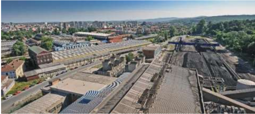
Figure 42. Panoramic view of the complex from the south side of the complex - view of the ash dump - part of zone 3.2 and part of the heating plant - zone 4.2 (close-up)
