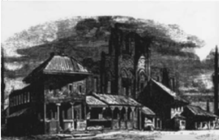
Plate 5.2 Precursors of the West: (a) The Wirtemberg barracks in Belgrade, 1736, built during Austrian rule; (b) the same building seen in 1864 as Pirinç-han (rice storehouse). Drawing by Felix Kanitz. ((a) From the plan of Nicola de Spar, 1736, reprinted on the CD ROM Stare karte, gravire i fotografije iz zbirke Muzeja grada Beograda , courtesy of the Muzej grada Beograda)
