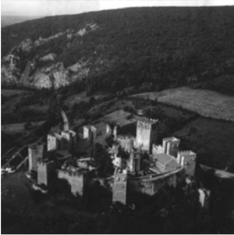
Plate 3.1 The church as fortress: Manasija (Resava) monastery, the endowment of Despot Stefan Lazarević, built 1407–17. (Photograph by B. Strugar)
