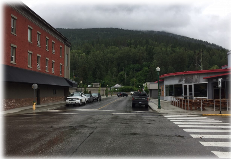
Orton Street Reconstruction Project
