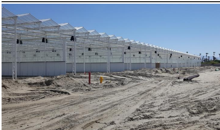
Figure 11: CPL greenhouse construction
