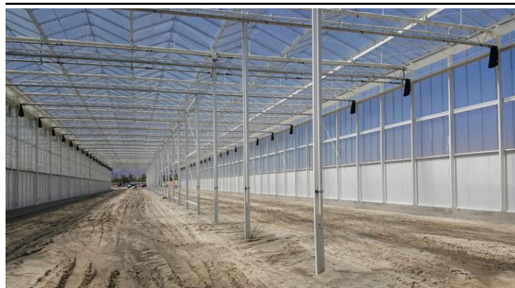
Figure 12: CPL greenhouse construction
