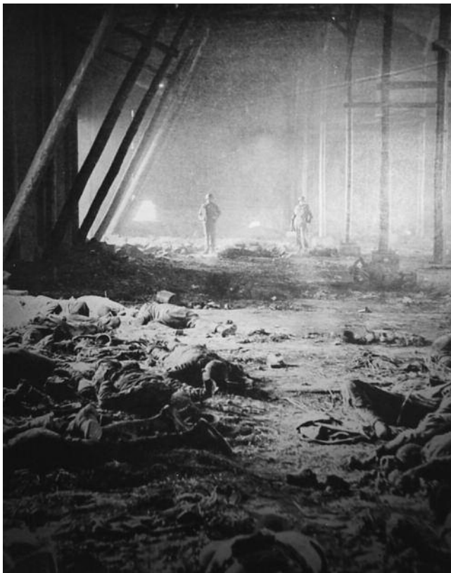
Left: The interior of the barn, looking down the long axis toward the west wall. This picture clearly shows the roof support posts up which Armand Dureux and others climbed to escape the flames and bullets. Note the hole in the far left
