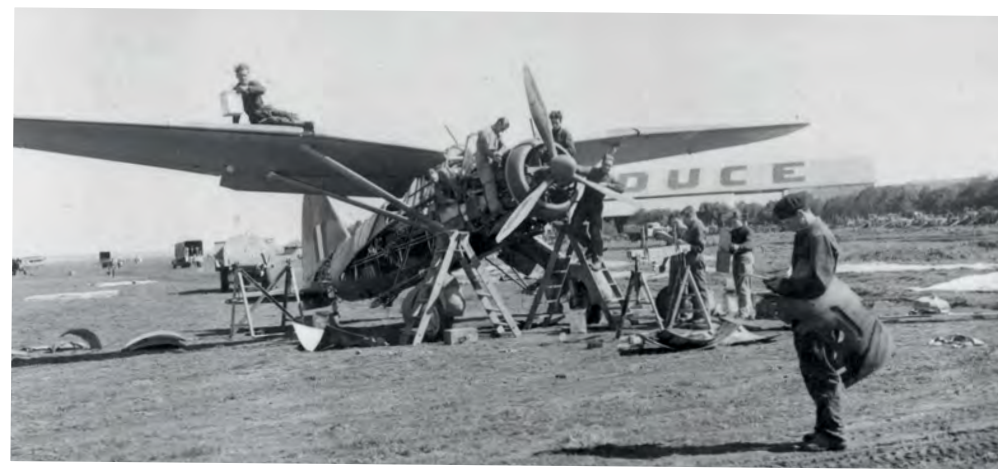
Above Maintenance on the former Italian airfield at Berce.
