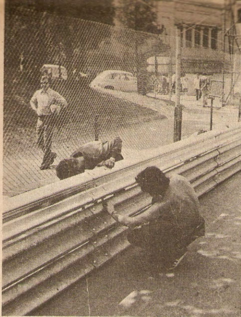
Mechanics fixing the guard rails in Spain . . .
