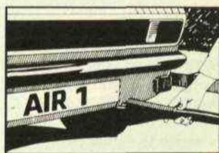
2. Fit cone securely over exhaust.
