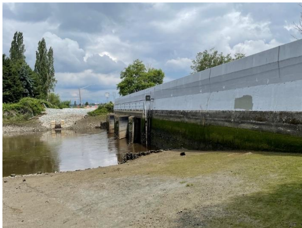
Existing Nicomekl water control structure (low tide, gates open)
