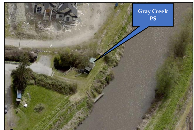
Aerial view of Gray Creek Drainage Pump Station
