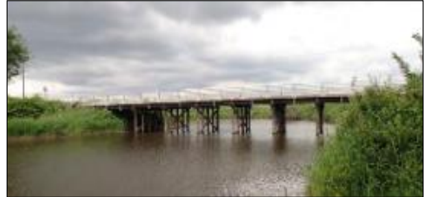
Bridge at low water showing aging timber piers and abutments
