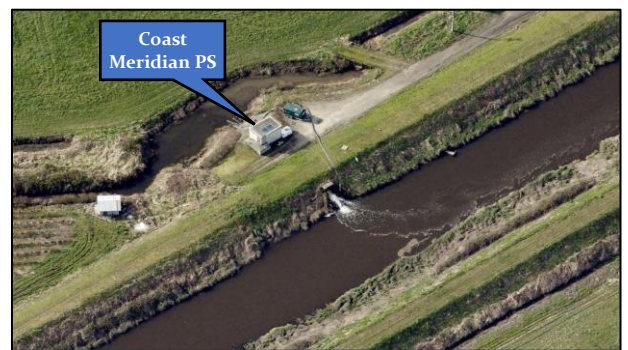
South facing view of Coastal Meridian PS draining into the Serpentine River
