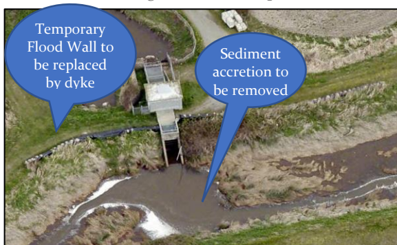
Existing Fleetwood Pump Station
