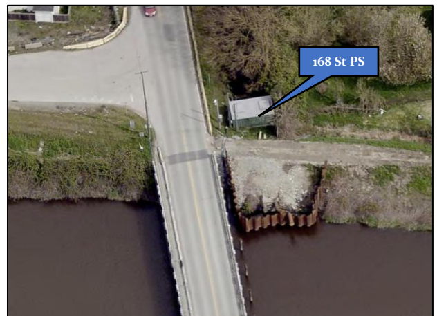
Aerial view of the 168 PS draining into the Nicomekl River
