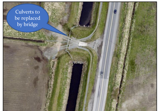
Existing 168 St North Canal 72 Ave Crossing
