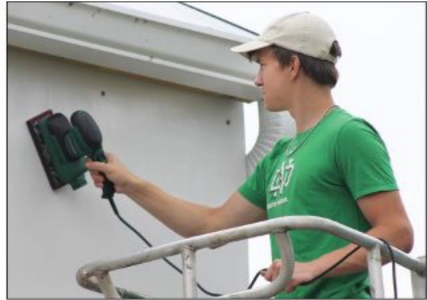
Ian McKay used a lift to reach the top of the building on Main Avenue with an electric sander. The surface needed to be sanded for the paint on the pending mural to grip to the surface of the canvas. McKay is one of several members of the Beta Theta Pi fraternity from Creighton University in Omaha, Neb. that came to town for service projects.
