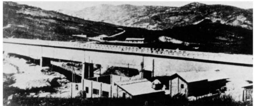
Only one picture was available to the planners of the raid and this was in fact 13 years old, having been taken in 1928 when the aqueduct was being built. The huts in the foreground used by the construction team were no longer there at the time of the raid. (Airborne Forces Museum)
