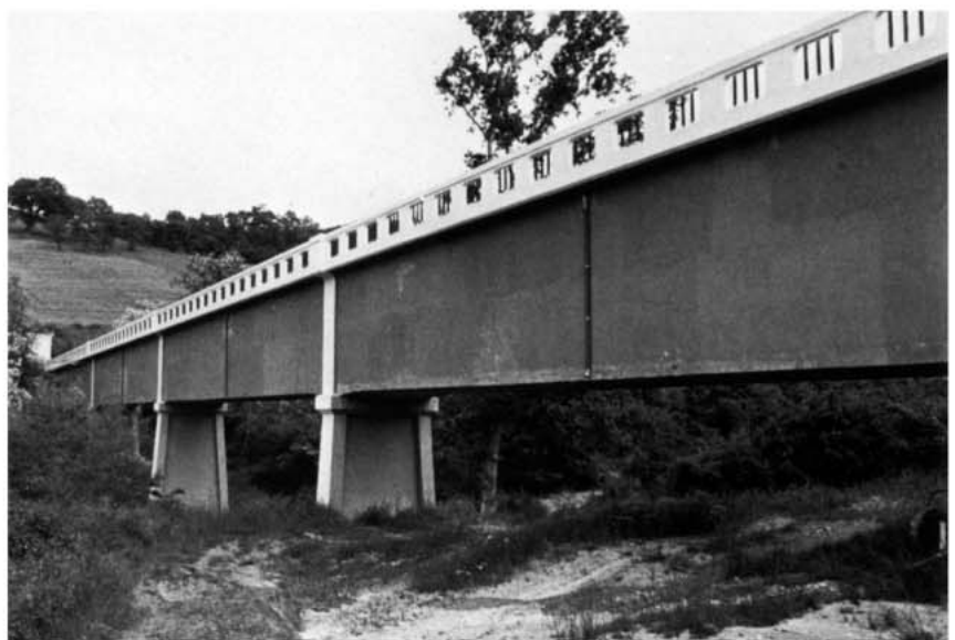
The demolition of the aqueduct was hampered by two unwelcome surprises: first, Lieutenant Paterson discovered that the aqueduct's piers were not of brick as they had been led to expect, but of concrete; then, with some containers missing and others impossible to find, it became clear that the amount of explosive available was much smaller than anticipated: only 800lb instead of the expected 2,240lb.
