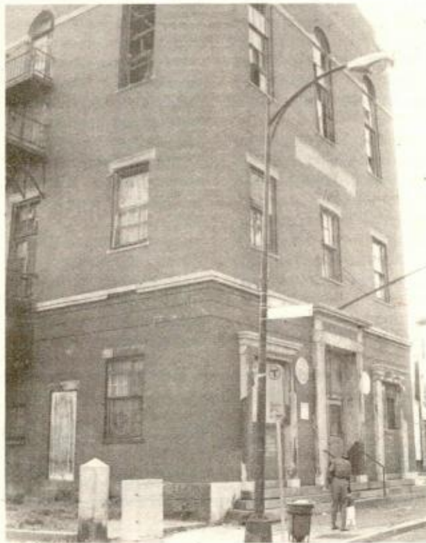
THE CHARLESTOWN MUNICIPAL BUILDING, located on Bunker Hill Street between Lexington and Ferrin streets, will be demolished before the end of 1991. (photo by Kathy Giordano)
