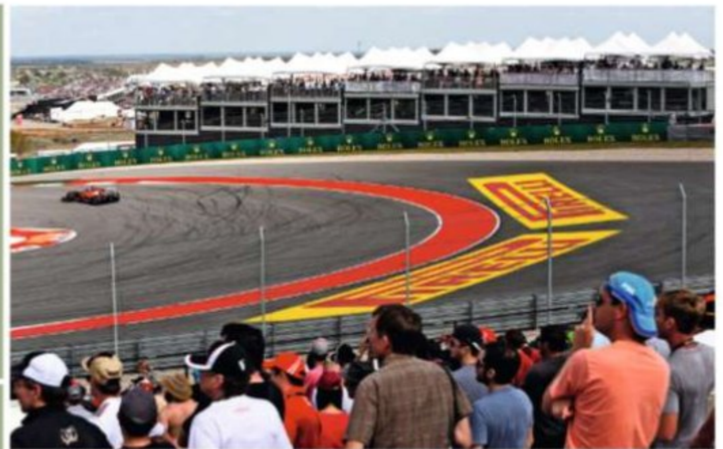
Turn 1 at Austin features the wide run-off areas that are now a feature of all modern Formula 1 circuits
