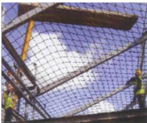
Figure 2.1 Safety nets on construction site. (Photo: Health and Safety Executive)
