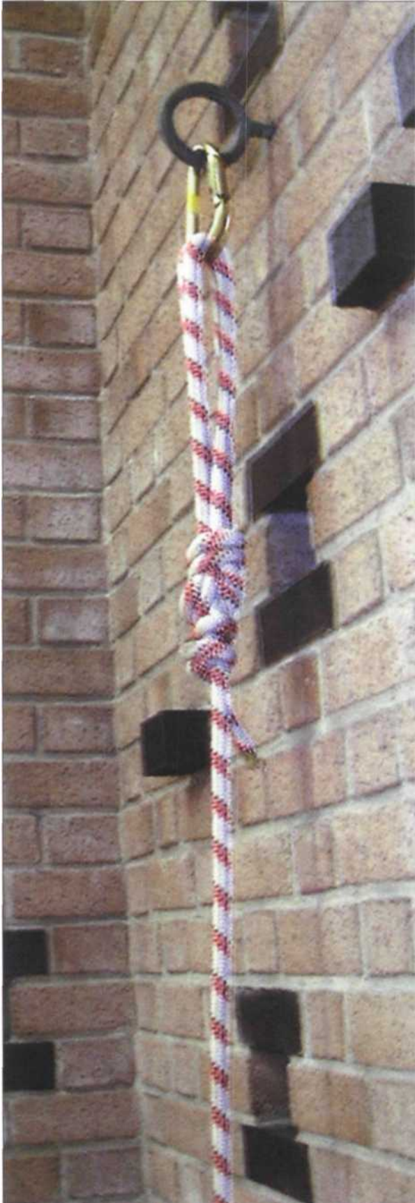
Figure 2.26 Photo of permanent artificial anchor.
